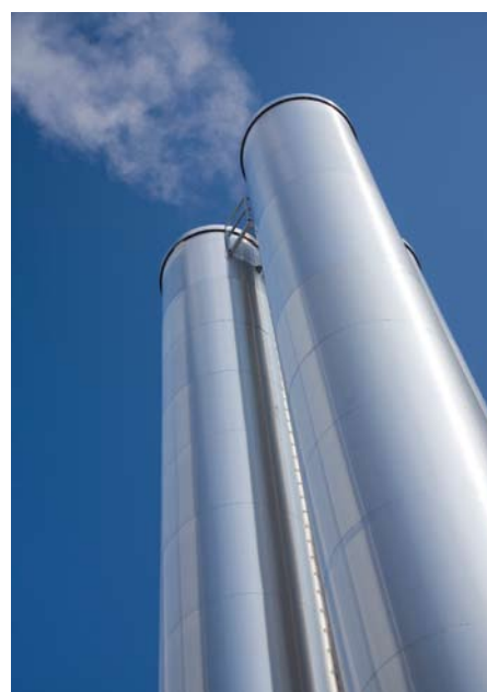
The new converters and acid plant reduce sulphur emissions from over 200 tonnes per day to less than 20 tonnes per day.
